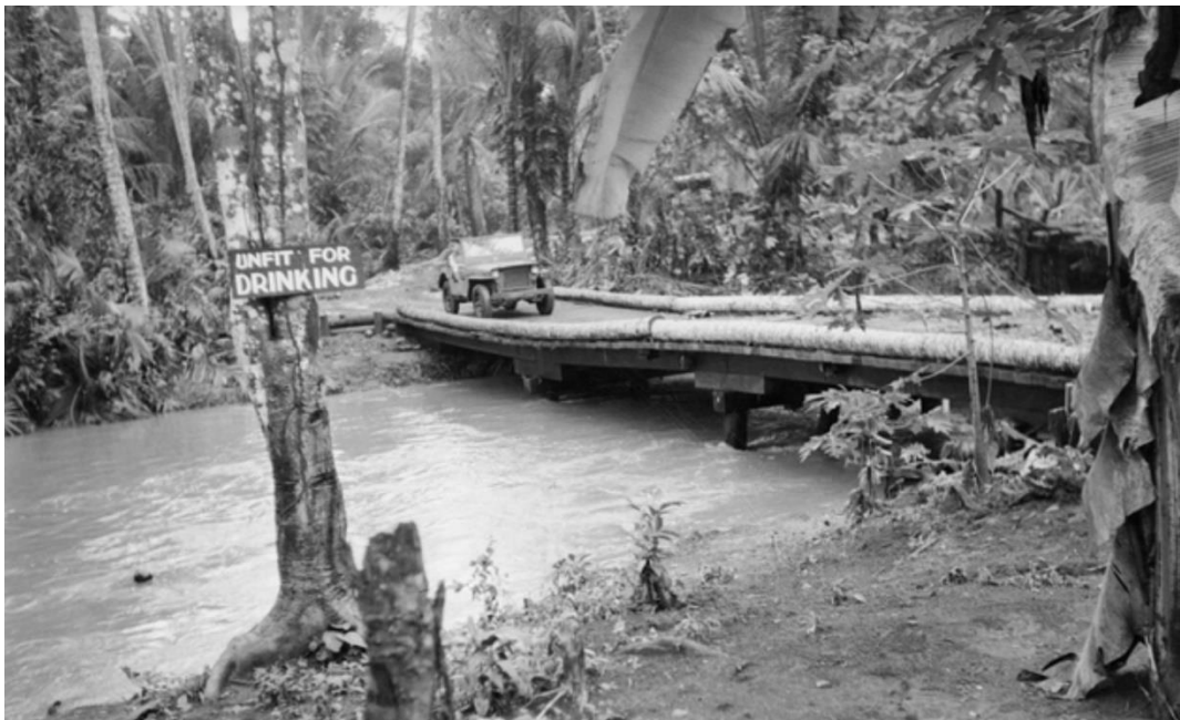
Milne Bay, Bridge Construction from coconut logs
